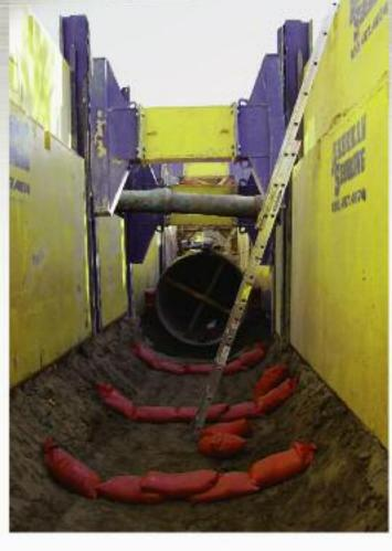
Vertical sheeting and trench support system for sewer, water, structure, foundations and soil remediation
